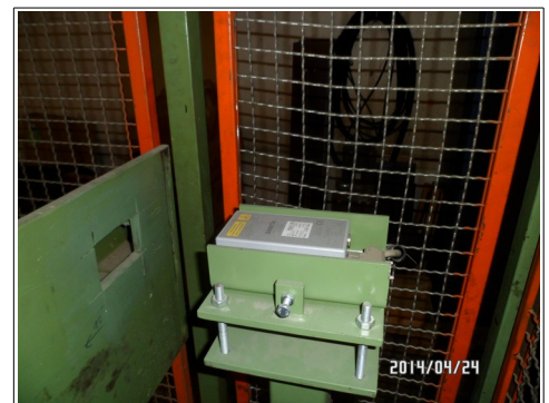
Pic 2: Installation of Sensor
